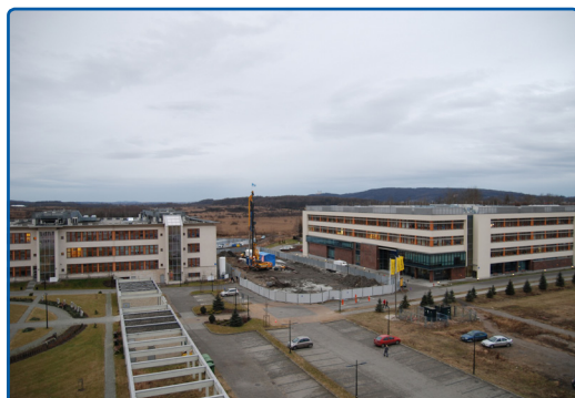
The construction site of Malopolska Center of Biotechnology
