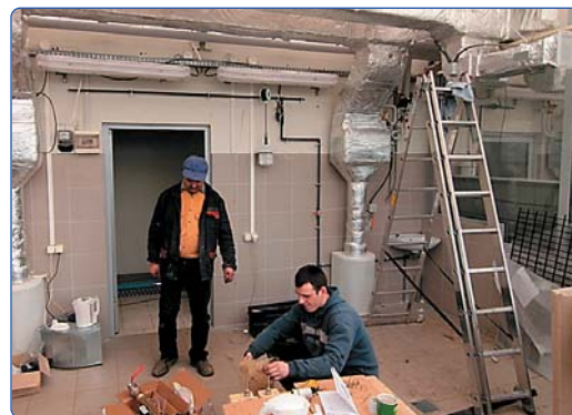
Modernising work in the greenhouse
